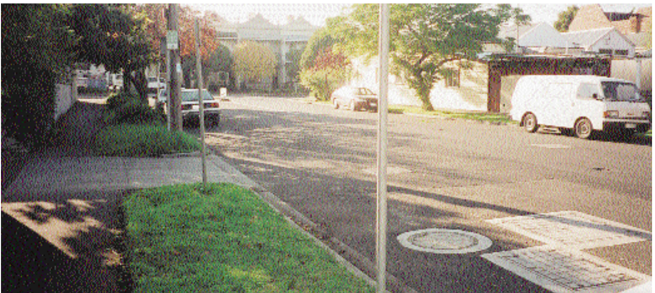
A typical Humegard™ installation in an urban streetscape - O'Grady Street, South Melbourne.
