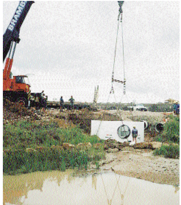
Humegard™ manufacture allows for installation in difficult site conditions including areas subject to tidal influence.
