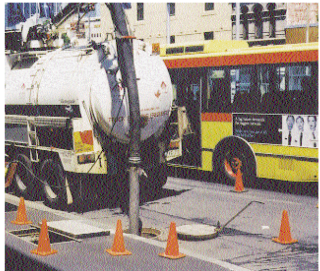
Maintenance of Humegard™ is carried out at surface level eliminating the need for confined space entry.
