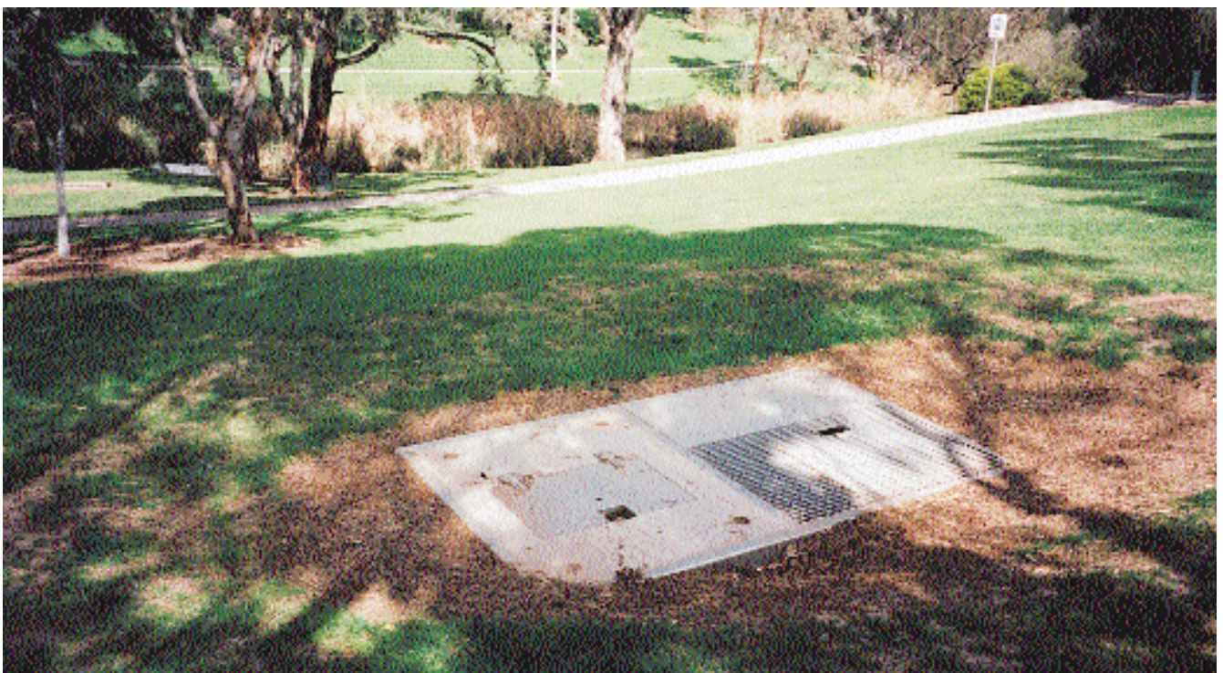
Humegard™ installation - Teatree Gully, South Australia.
