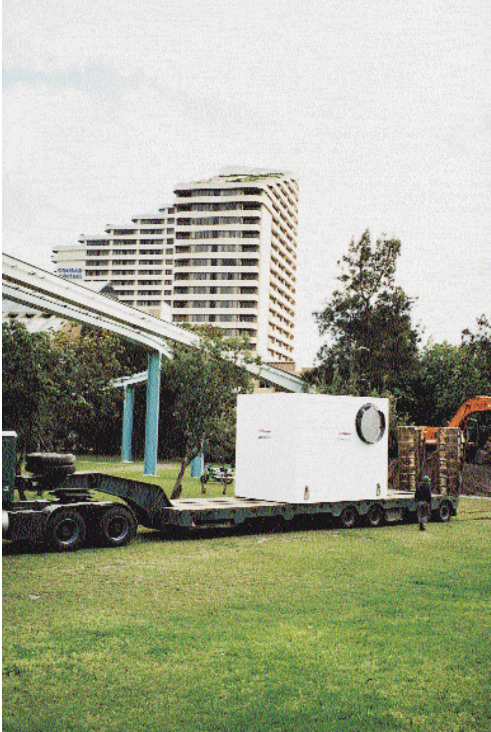
Humegard™ installation for tidal application - Broadbeach, South East Queensland.
