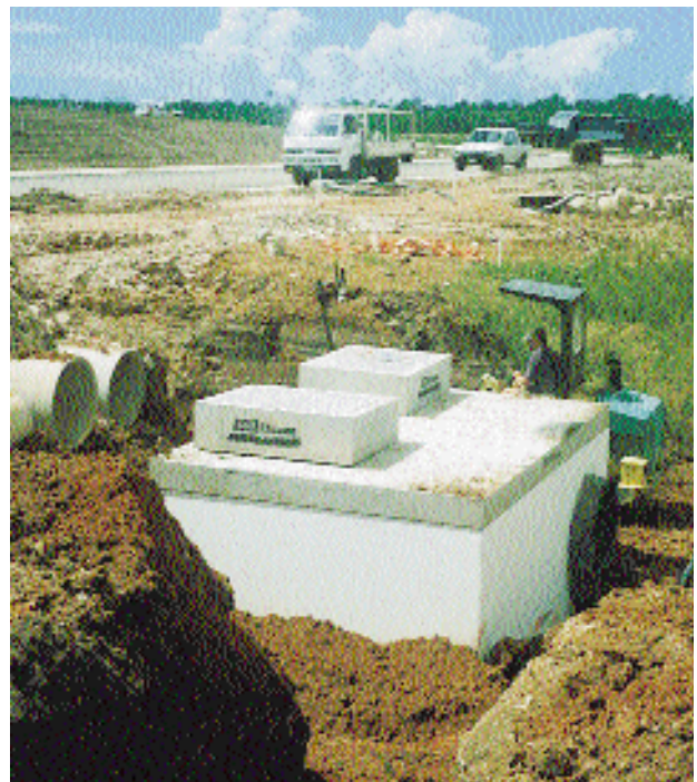
Located in the stormwater drainage system - Humegard™ does not require difference in elevation between the inlet and outlet invert of the pipeline.
