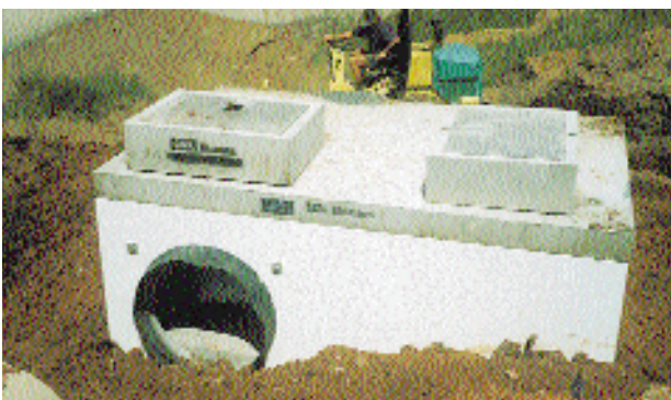
Construction with precast components allows for immediate backfilling once the Humegard™ has been positioned in place.
